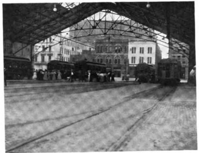
TRAIN SHED, INTERURBAN UNION STATION, INDIANAPOLIS
